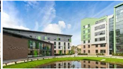
GWP Architecture, "The Green", Bradford (UK), 2012 ©GWP *BREEAM - punteggio 95.05%
